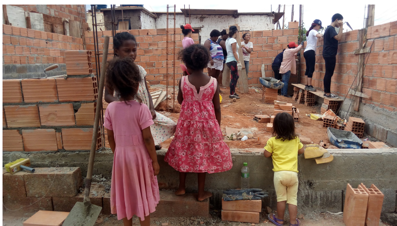
Figure 6. Construction workshop for women in the Rosa Leão Occupation
