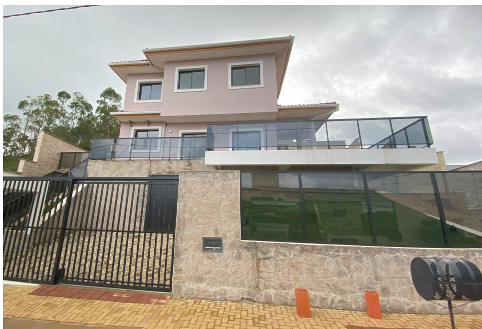
Figure 8. House nearing completion in the Bento Rodrigues resettlement (2022)
