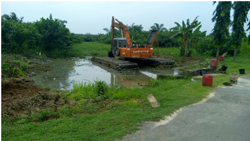
Figure 8. Desilting/Dredging works along a flooded waterway while heavy rain is still at its peak (photo taken in May 2023)
